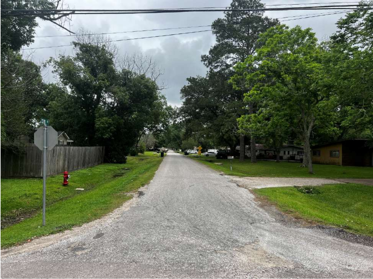
Picture 11: Looking east down 24 th Street from where it intersects with Avenue M.
